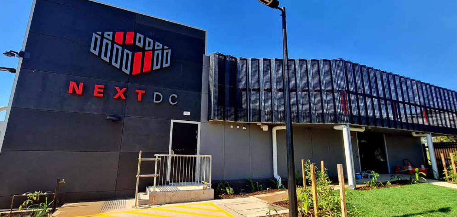
NEXTDC D1 data centre in Darwin.
